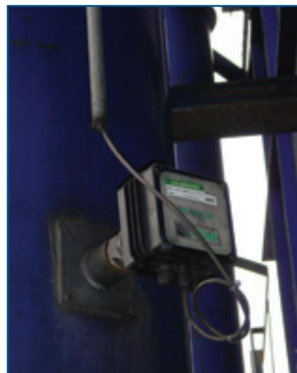
*Electrodynamic® Sensor installed in bag house outlet*
