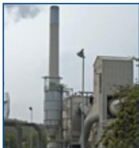
A Cement Kiln Baghouse incorporating an Electrodynamic® filter management system
